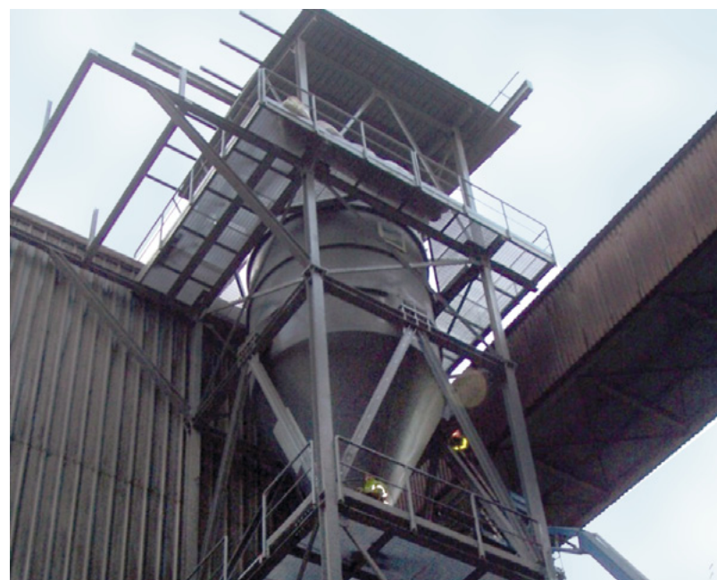
Steel Meltshop Vacuum Degassing Bag Filter (Europe)
