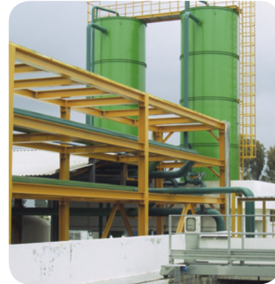
Sludge thickeners
